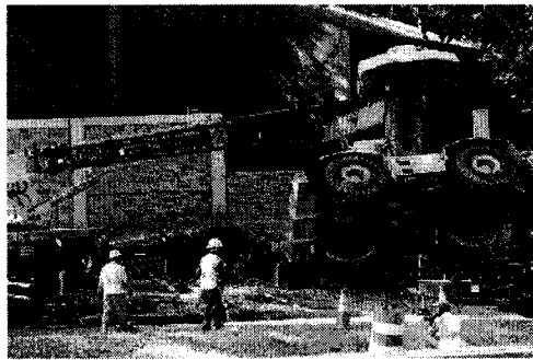
This crane tipped over near Shady Grove and I-370.
