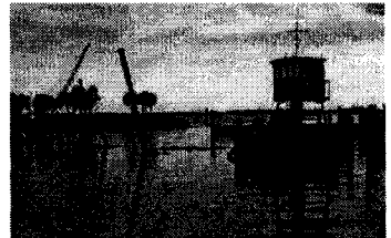
A barge holding crane sank today at Titusville Municipal Marina. About 100 gallons of diesel fuel were spilled into the water. (Malcolm Denmark, FLORIDA TODAY)
